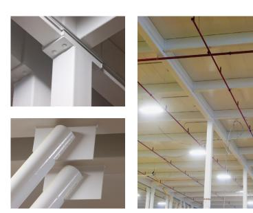
Alternatives to HSS were considered, but resulted in high fabrication costs compared to HSS.
