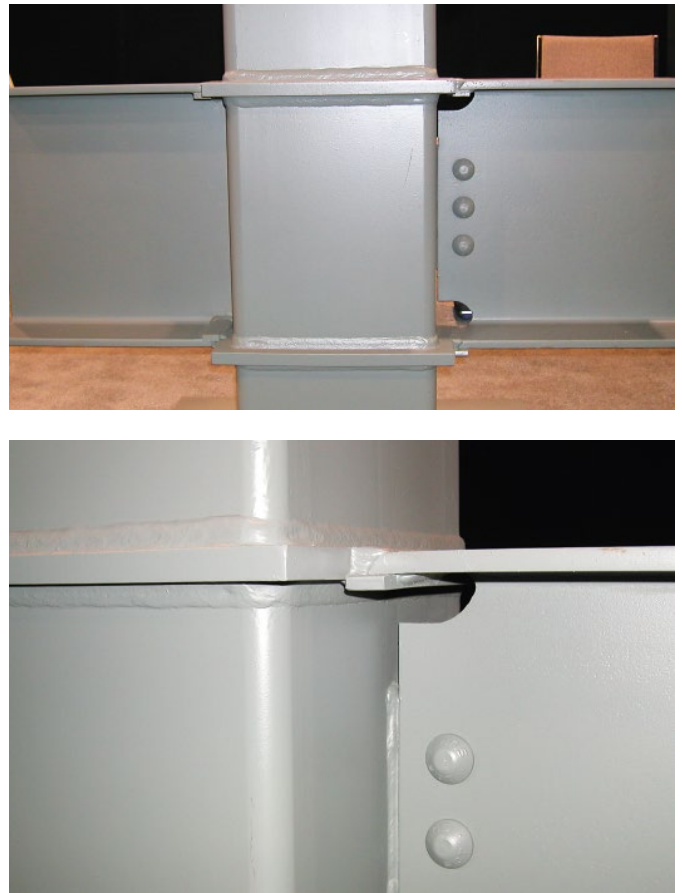
Fig. 4. Welded through diaphragm connections, commonly used in Japan, to cold-formed RHS columns
