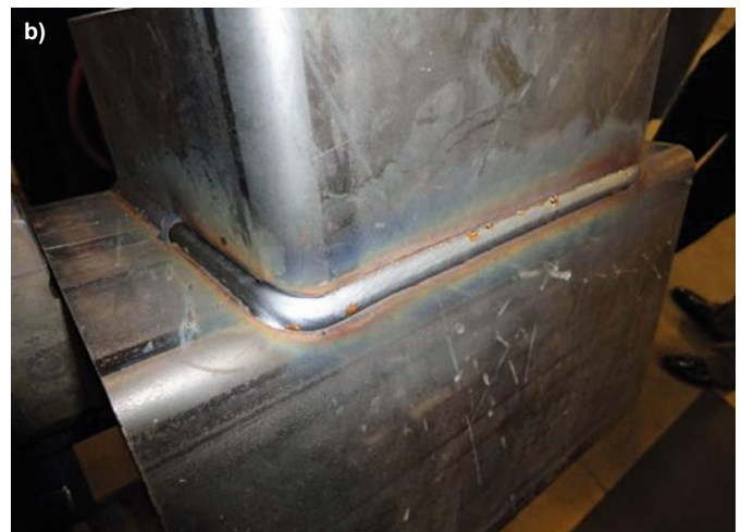
Fig. 2. Cold-formed RHS members welded in the corner regions: (a) cross-section of flare groove welding; (b) matched width T-joint
