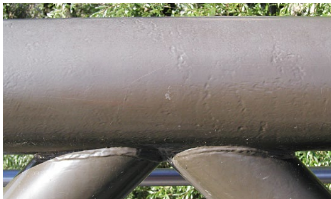
Fig. 1. Hollow structural section bridge truss, with a close-up view of the surface finish on the hot-finished chord member
