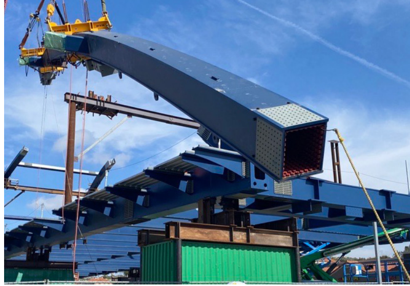
An arch rib with Shuriken being lifted into place. Walsh prepared complex rigging to lift the tilted arch ribs in the proper orientation.
