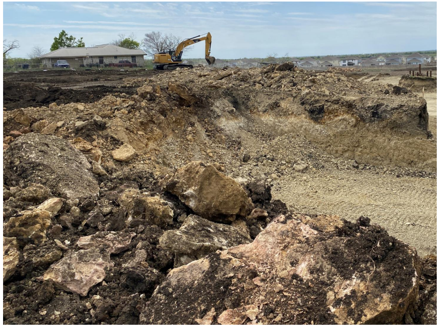
Jarrell – Surface Rock Not Found in Geotechnical Borings.
