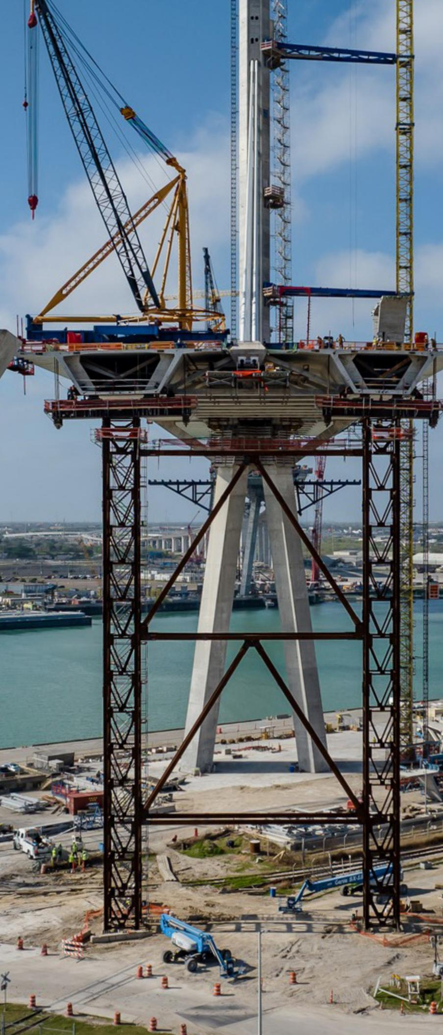
and field bolt the supports on-site. This saved ATS time and money on procurement, logistics, and fabrication. “I was able to save money by buying in-stock material instead of mill-run material,” says Lee. By purchasing standard lengths, ATS cut lead time by several weeks and was able to transport the braces to the site without the need for an oversized load designation, reducing freight costs.
