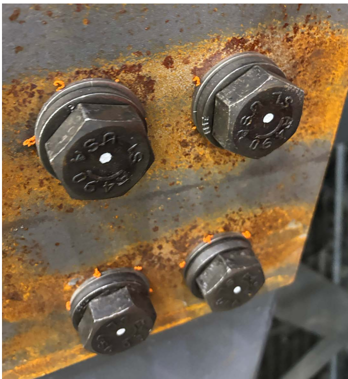
Fully pretensioned 1" A490 bolts installed with DuraSquirt DTI's for fast visual inspection. Shuriken is the only way to install large, slip-critical bolts from one side.
