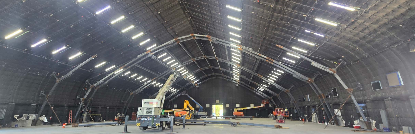
A frame being erected. The end sections have been set, and the center section is assembled on the ground. The interior space meant all lifting was done with a small crane.
